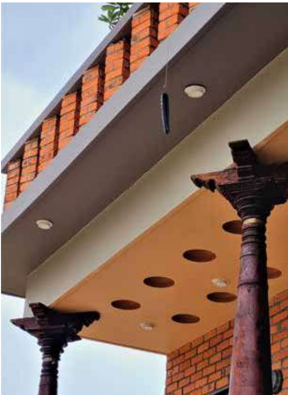
Filler slab having green slab just above it, Chettinad Pillars & Louvered parapet to provide fresh air and day light to the green slab above and to dining kitchen
